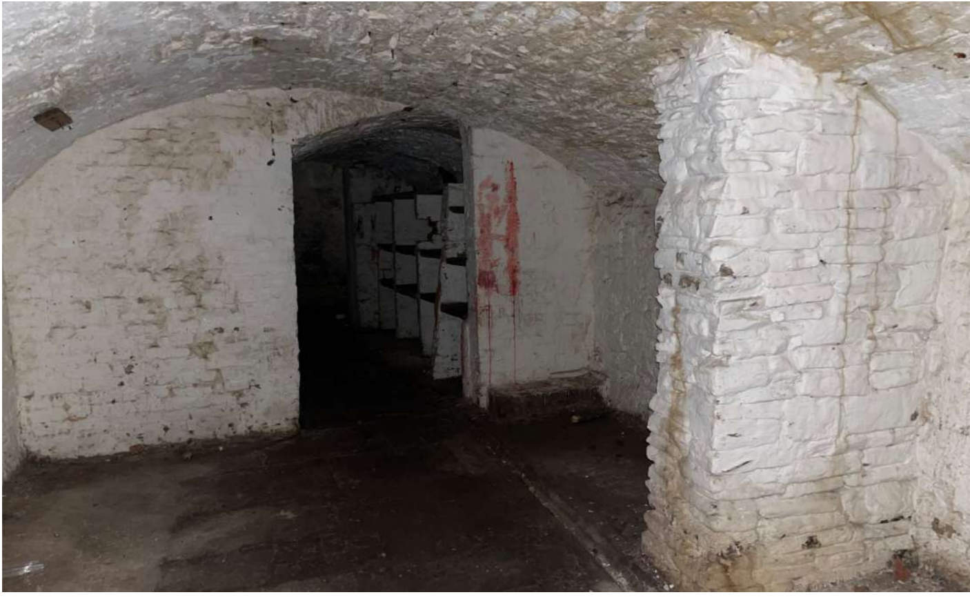
Internal view of the existing cellars.
